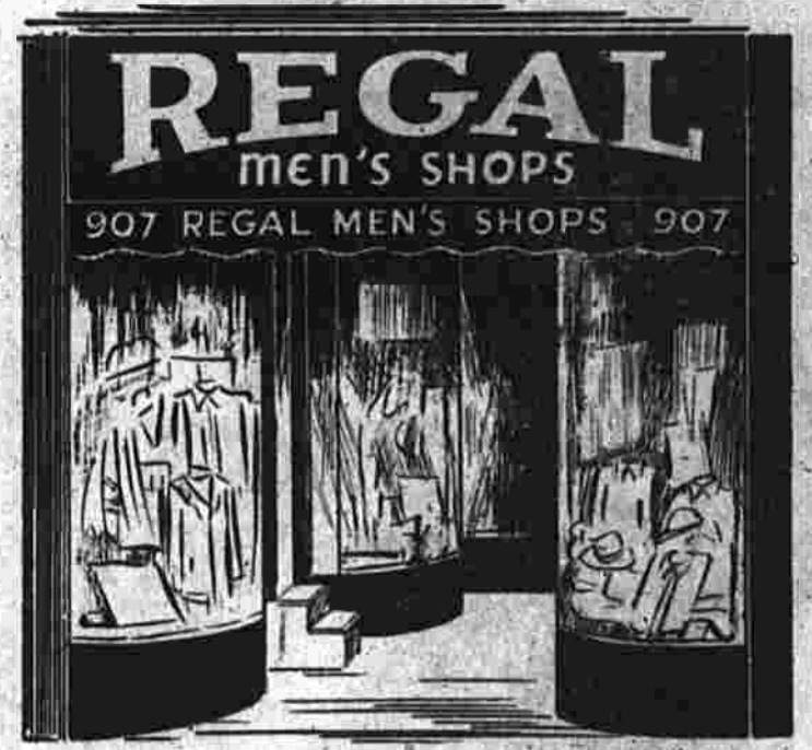
Photo above of the old Regal store front bears out the old saying "Big odds from little odds grow" when you take a look at the new front pictured at left. It bears out the fact, too, that the size of a store isn't nearly as important as what goes on inside. And the pleasant customer relationships that went on inside this small store are what led eventually to great transformation at Regal Men's Shop.
